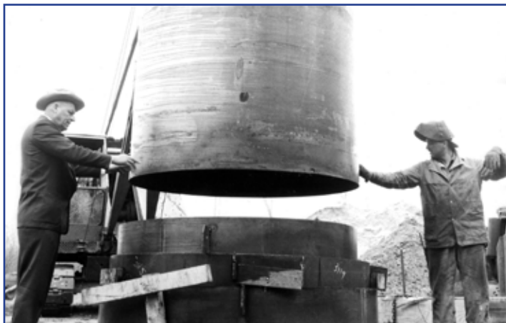
This is Frank J. Haupt and my eldest brother Sylvester in the process of setting caissons.
