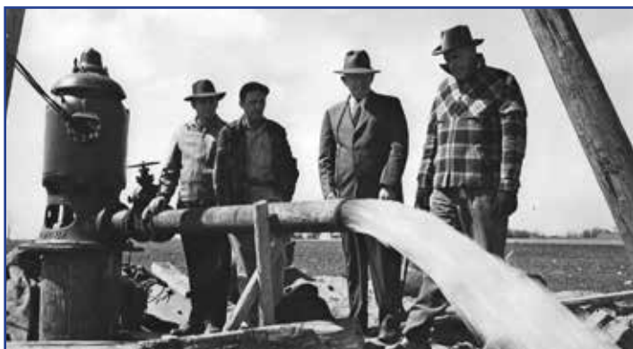
Frank, a gentleman from the City of Marshfield, and others checking the flow of a recently constructed caisson well (note the large wood pole tripod used for construction).
