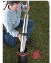
test confirmed the pump was hitting the curve, Dan asked the customer for more information about the discharge piping. The customer recently purchased the property and had limited knowledge of the piping. While the customer started digging, Dan continued to review the numbers.
